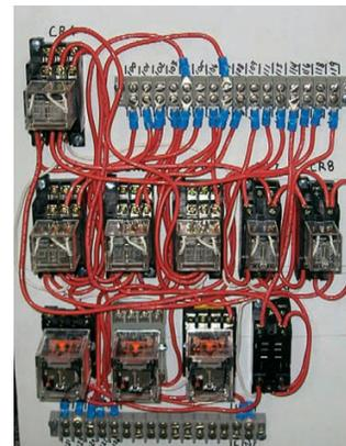
(a) Relay-based Control Panel
