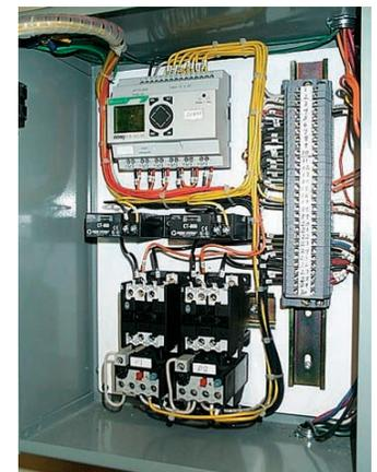
(b) PLC-based Control Panel
