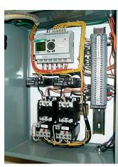
(b) PLC-based Control Panel
